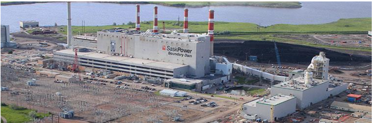
Fig 1. The Canadian Boundary Dam Power Station using carbon capture and storage technology.
